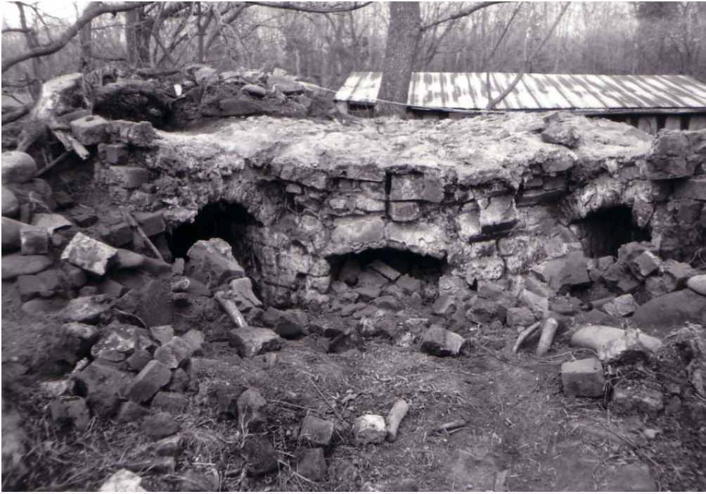
Exterior of kiln, looking north, March 2000, after cleaning and gridding. Dome and chimney long since removed, but interior chambers are intact.
