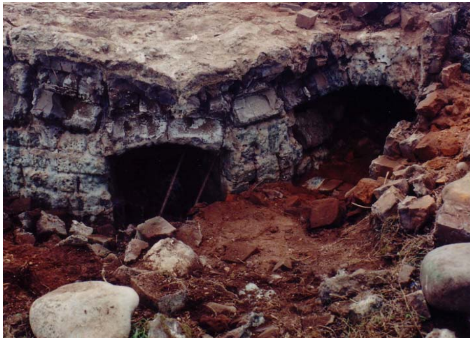
Exterior of kiln, looking north, March 2000. Thick glaze on bricks; central chamber (fire box?) opening propped up with iron rods.
